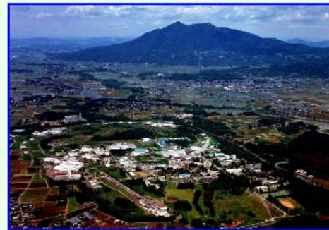
The KEK site is located close to the Mt. Tsukuba, about 70 km from the both Narita-Tokyo airport and central Tokyo. This picture shows the 400 m long electron and positron linac and the buildings above the collider ring, whose circumference is about 3 km.
